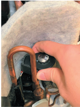
Remove the EEV coil by hand.
