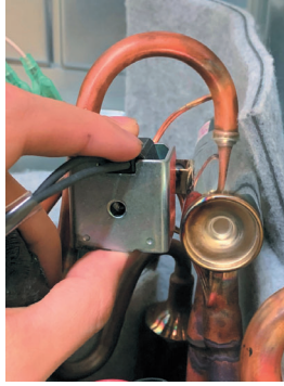
Remove the SOLENOID COIL
